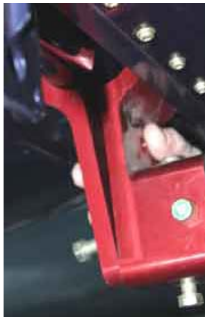
Figure 10 View Showing the Installation of the G2-1 Cross Tube Bracket
